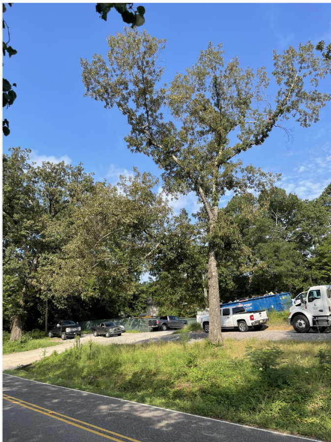
3 TREE REMOVAL ALONG MASSEY - A
