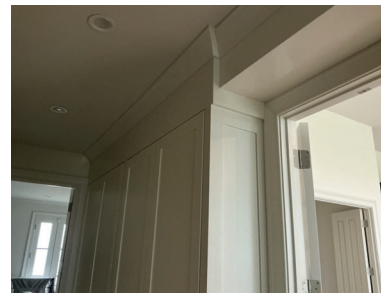
TYPICAL BUILT-IN CABINERY AND CROWN MOLDING
